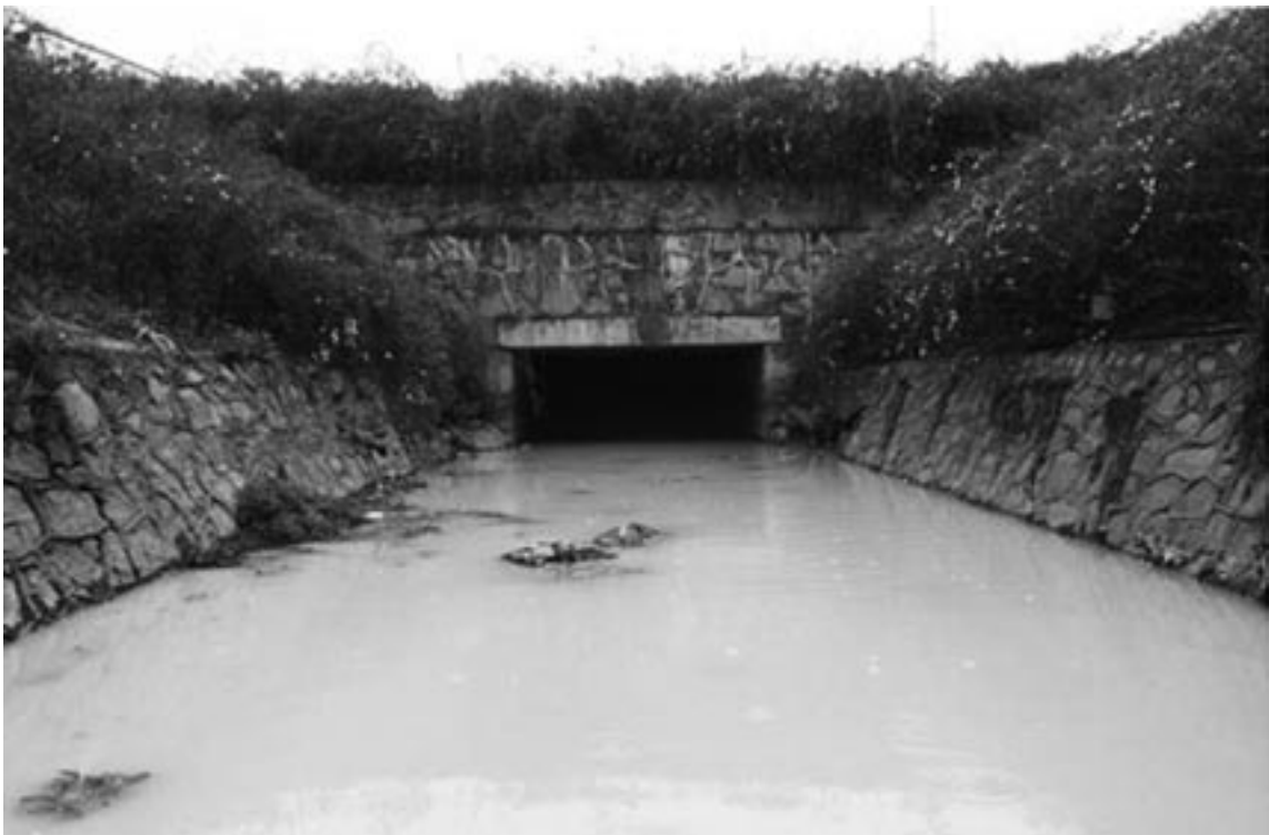
Discharge Channel Leading to Nantaizi Lake near to Wuhan's Meiko Electronics (Photo: Ma Jun)
