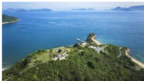
Aerial view of Benesse House
