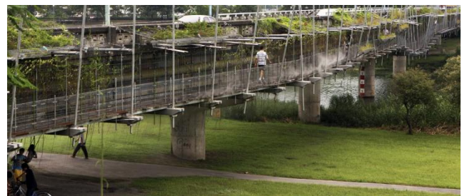
Jin-Mei Parasitic Pedestrian Pathway across Yilan River © Fieldoffice Architects
