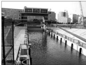
This recently completed lock system in Tokyo connects the Arakawa River with the old canals of the Koto Delta, such as the Nakagawa, shown here. Because the Arakawa is tidal, its water level fluctuates with the ocean; meanwhile, the streams of the Koto are kept lower than sea level to prevent them from flooding the neighborhoods they crisscross.
