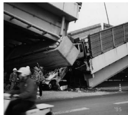
Picture 1 Collapse of the Hanshin Expressway Route 3 (Kobe Route)
